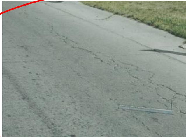
% surface area with fatigue cracking
